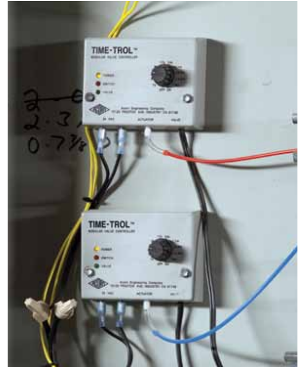
Time-Trol® valves may be located near the fixtures or at a central location up to 100 feet away.
