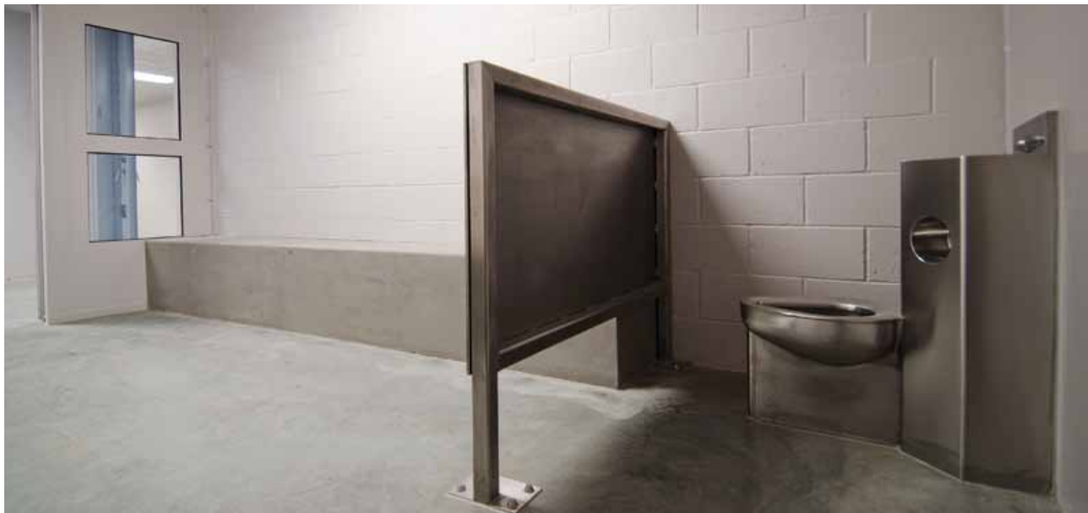
On-floor, 18-inch Penal-Ware® Comby withstands 5,000 pounds of force without permanent deformation (1418-CT-2-BPH-04-M-FV-PHRF-SPS).
